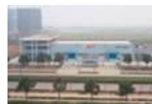
Suzhou, China Level, Pressure, Flow
