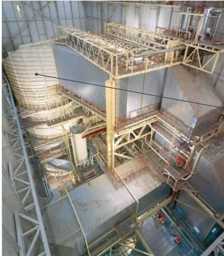
Washing tower of the flue gas desulphurization absorber
