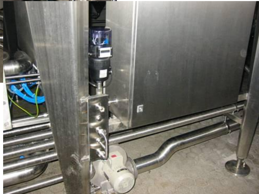
Valve node (Platomass outlet)
