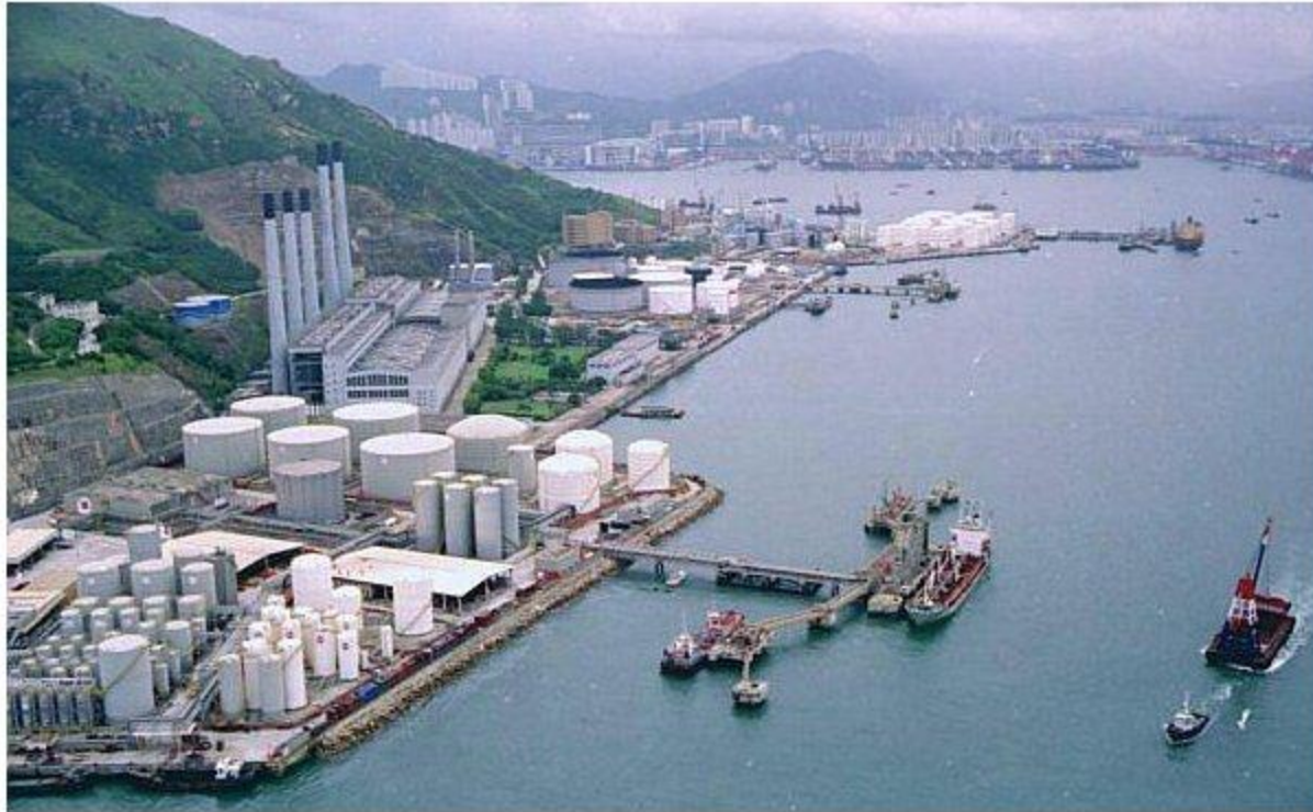
Three tanker terminals for oil depots at South Tsing Yi
