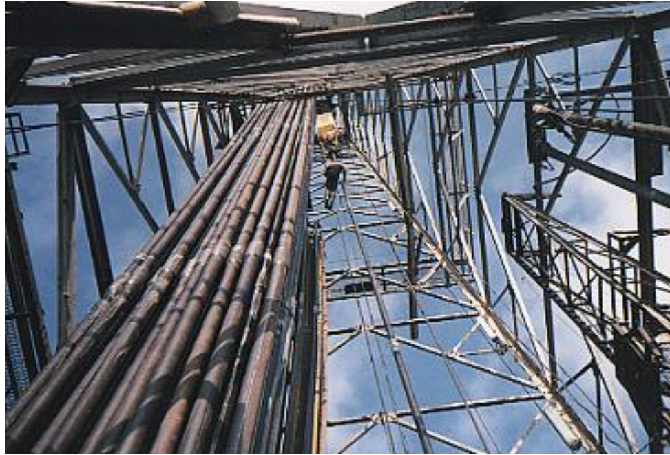
The stands are placed for future use in the derrick.
