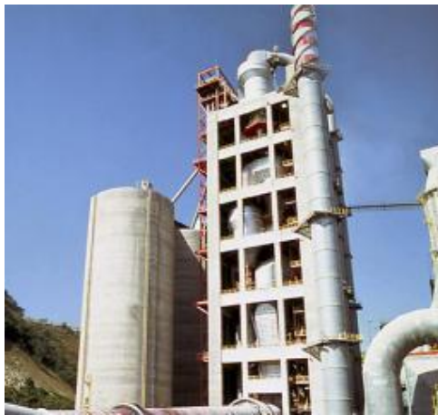
Clinker silos / Coal bunker
