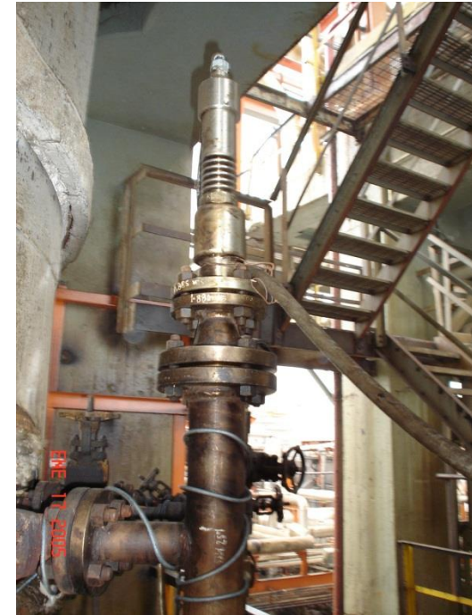
Installation of the Levelflex FMP 45 in the high vacuum tower
