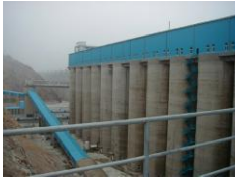
Grain silos / Bulk storage
