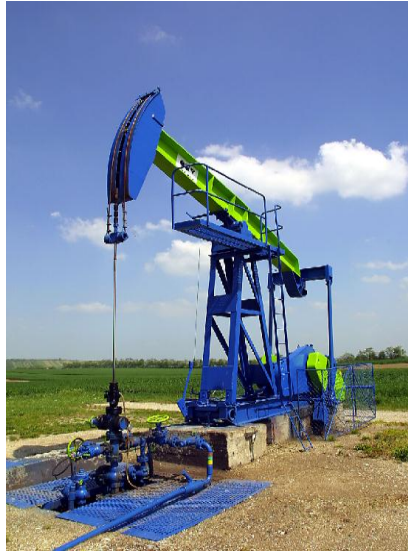
OMV wellhead and pump
