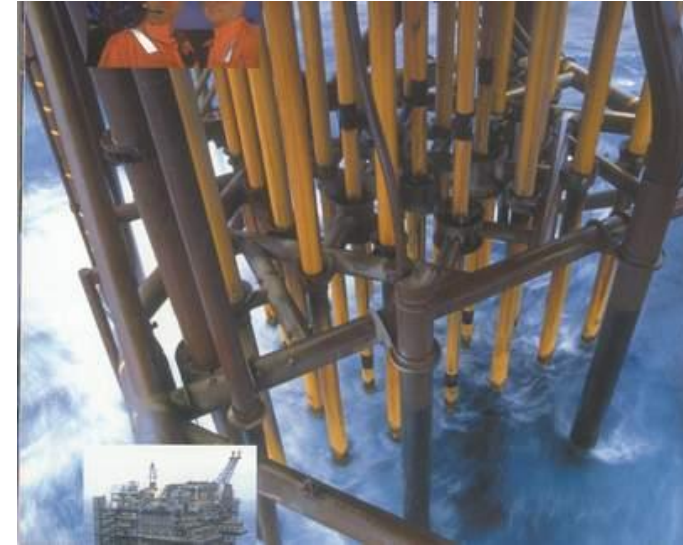
Cluster of risers of a FP, fixed platform
